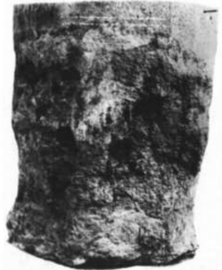
PLATE 9.4 The bottom part of one of the sandstone columns, Buhen temple, Sudan. This illustrates the flaking away of the surface layer due to efflorescence
